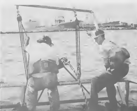
LAUNCH WORKERS lower the rake which is attached to 100 feet of heavy three-inch line. The rake is pulled at a speed of four knots. TRAHADORNAN DI lancha ta baha e halakó cu ta mará na 100 pia di cuba di tres dun y mitar.
